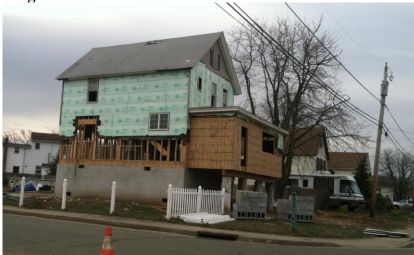
Figure 19: A home is raised at Dock and Second Streets.
