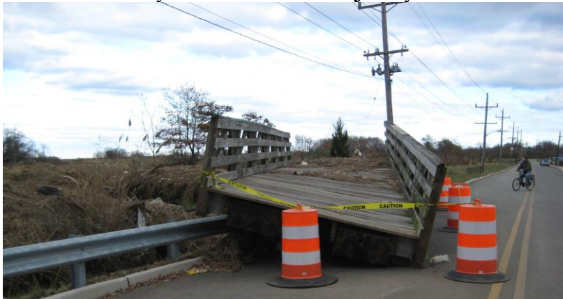
Figure 12: Superstorm Sandy relocated a foot bridge from the Henry Hudson Trail onto Jersey Avenue.
