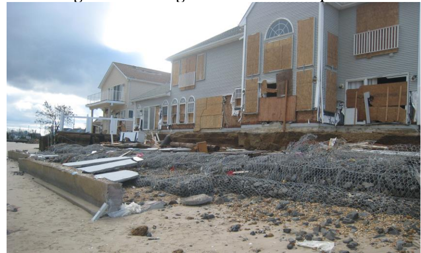
Figure 17: Damage to Beachfront Properties
