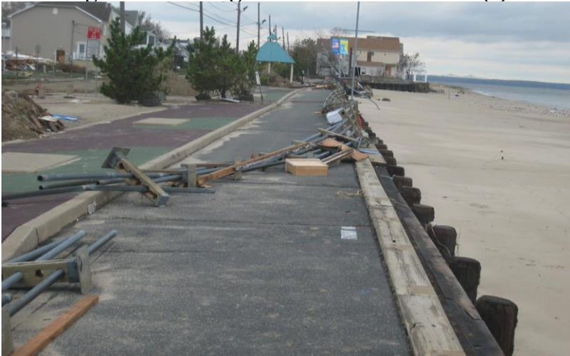
Figure 16: Damage to the Shorefront Area (2)
